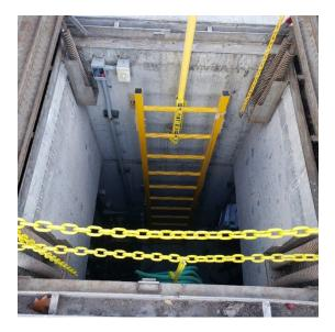
The vault has a ventilation system that blows fresh air into the vault at all times, however atmospheric monitoring will take place prior to entry and the confined space classification checklist will need to be completed prior to entrance into the vault (Appendix A). This checklist will be used to determine if the space can be declassified to a non-permit confined space and be entered using alternate procedures. Alternate procedures can be used to enter the space when:
